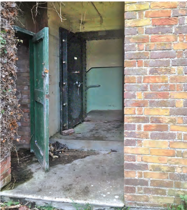
The entrance to the bunker at the rear of the walled garden. The first door is a store room with the gas-tight door into the bunker beyond. Photo Nicholas Gould
